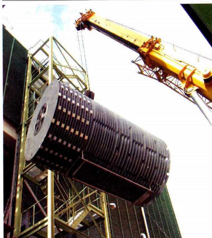
Lifting the new agitator of the finisher
